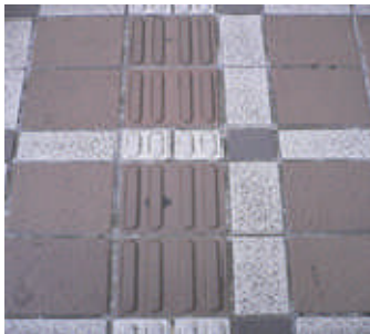
Fig. 1 An example of TWSIs with low visibility.
